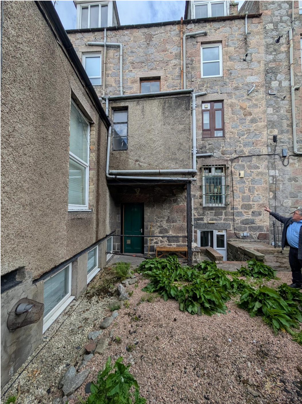
Fig. 4 – Rear elevation showing washhouse/toilet block in relation to main granite building.
